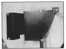
**STEP 34**Place four Speed Clips on the Amplifier Bracket as shown.
